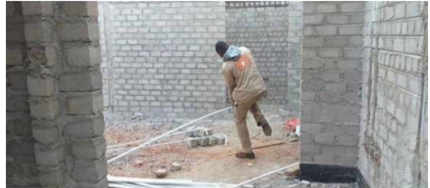
Fig 7. Construction progress- subcontractor working on first fixes for electric works
