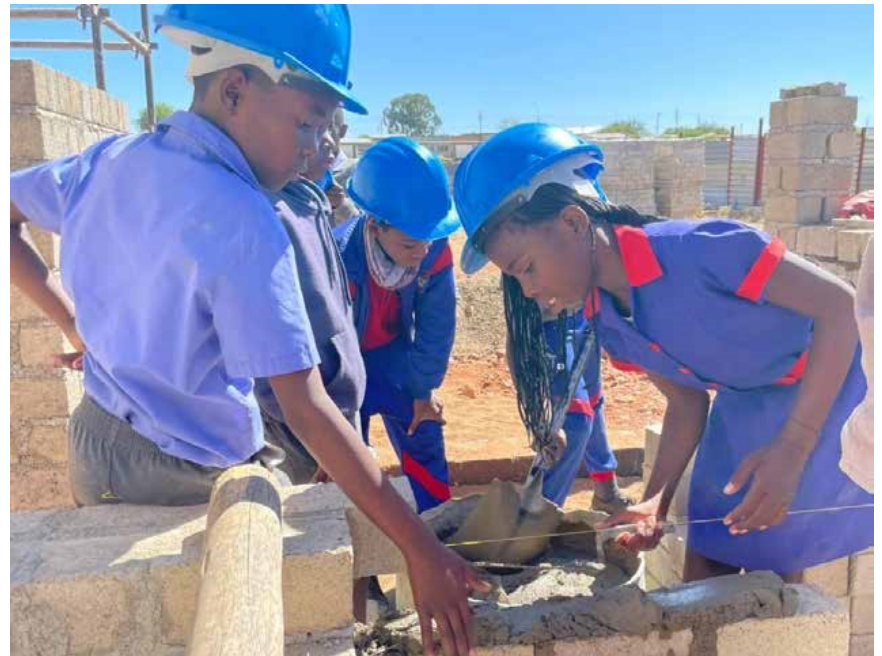
Fig 20. Community Engagement- St Barnabas, students participating in bricklaying and cement mixing
