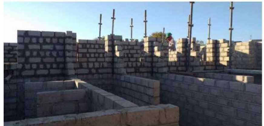
Fig 7.1 Construction progress- erection of building superstructure
