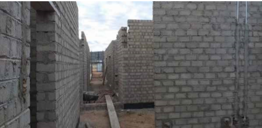
Fig 10. Construction progress- view of internal passage
