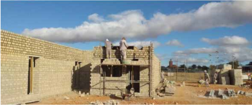
Fig 8. Construction progress- erection of superstructure to ring beam height
