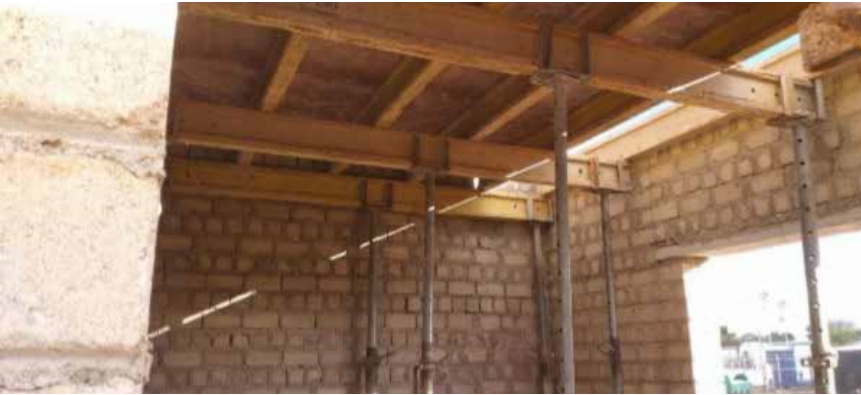
Fig 9. Construction progress- erection of form work of concrete roof slab
