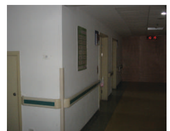
Pict.50 Protection wall floors (new construction)
