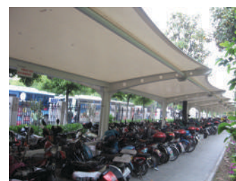
Pict.4 bicycle parking facilities
