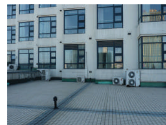
Pict.12 Facade wards
