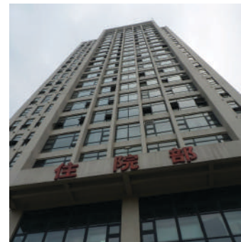
Pict.56 Open windows ward building (new construction)
