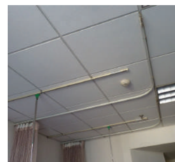
Pict.19 Ceiling Patientroom (new construction)
