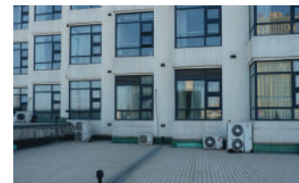
Pict.14 Facade wards
