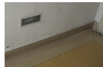
Pict.16 Flooring wards (new building)
