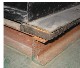
Pict.20 Decoupling technical equipment
