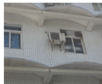
Pict.8 Fassade ambulance
