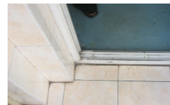
Pict.31 Threshold Toilet Patientrooms
