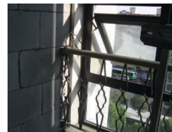
Pict.21 Handrail patientrooms ward (new construction)
