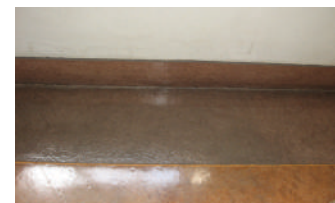
Pict.17 Flooring wards (old building)
